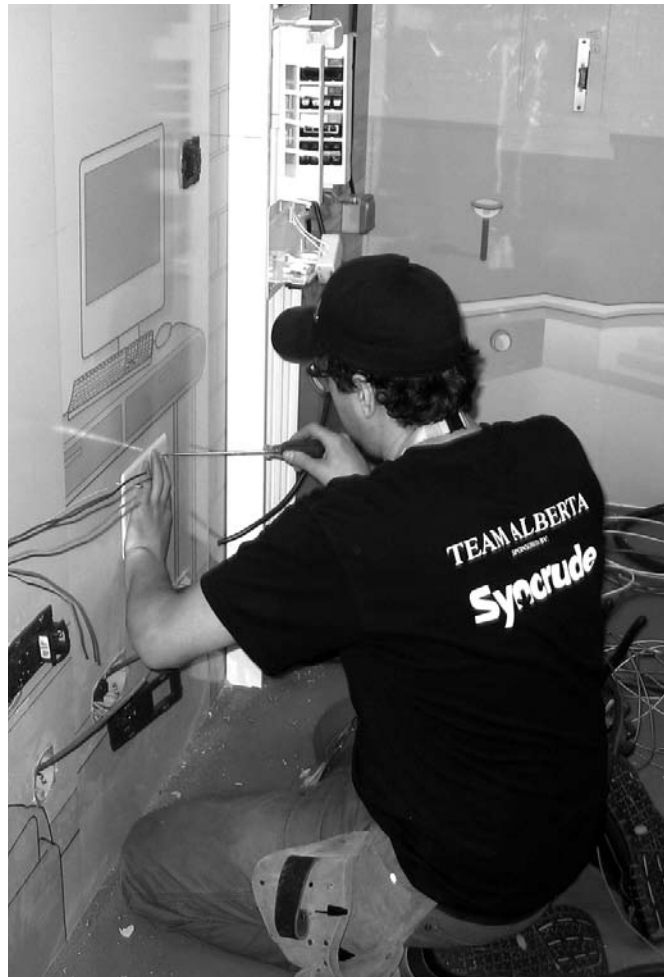
Craig Spady, 2009 Team Canada Electrical Installations
